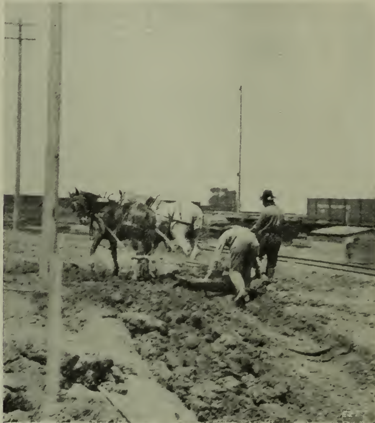
FIG. 1. DRAG SCRAPER IN USE.
